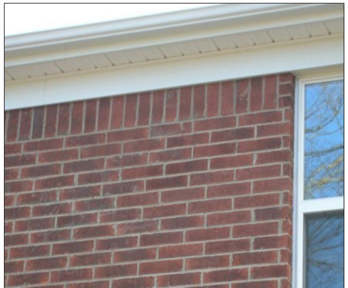
**Photos 1 and 2:** Before staining (top), lighter-color brick stands out. After staining (bottom), they blend with the surrounding brick.
