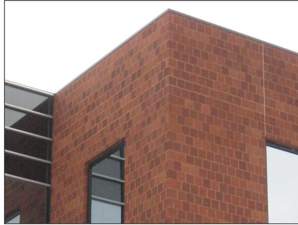
**Photos 11 and 12:** Before staining (left), all the brick units were the same color. Brick staining was applied to certain individual brick units to create a variegated appearance (right).
