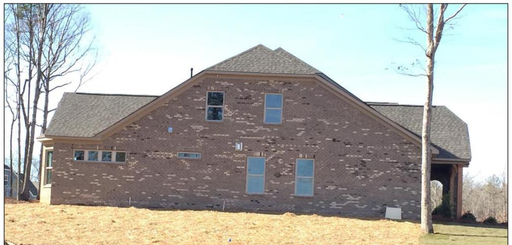
**Photos 5 and 6:** Before staining (top), brick from different production runs were installed, causing inconsistent color. After staining (bottom), the facade had a well-balanced blend of varying brick colors.
